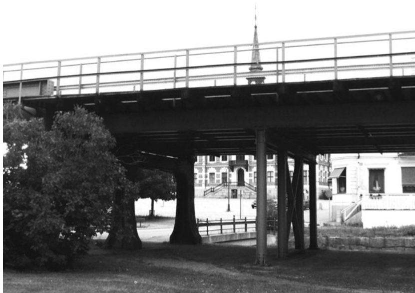
Figure 1. Railway viaduct adjacent to the town hall in Söderhamn. Photo: Krister Olsson (2005)
