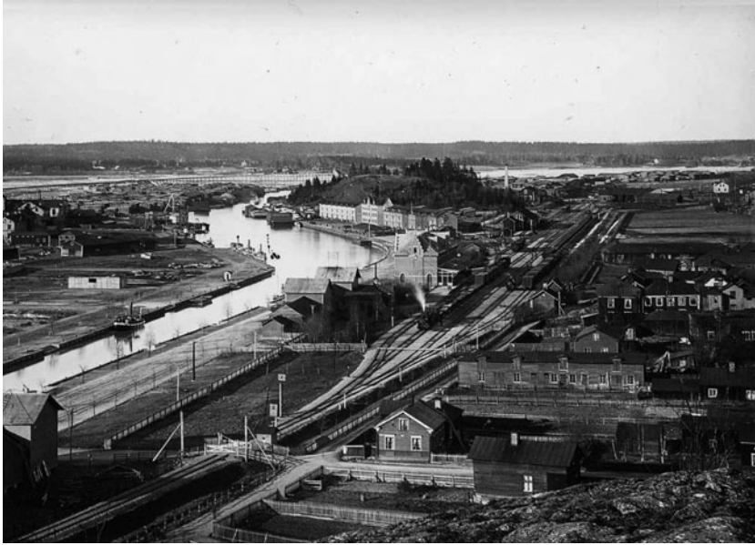
Figure 3. Söderhamn, the marshalling yard and railway station in 1900. Photo: Nybergsska samlingen, Sveriges Järnvägsmuseum, Gävle. Courtesy of (CC) Michael Lindgren (2008)
