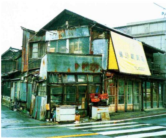
Figure 6: Bad Condition Traditional Building along Katori Street in 1980s
