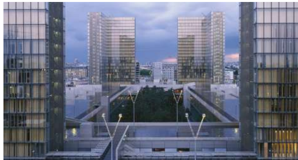
▲ NATIONAL LIBRARY OF FRANCE(Paris, France) https://www.perraultarchitecture.com/en/homepage/
